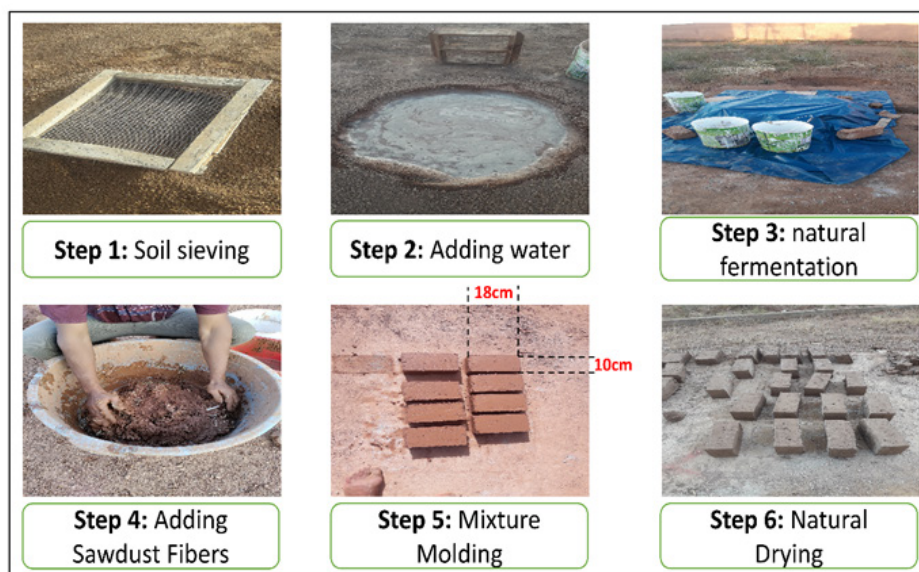
Figure 3: Process of Adobe Brick Preparation[39][40][12]
